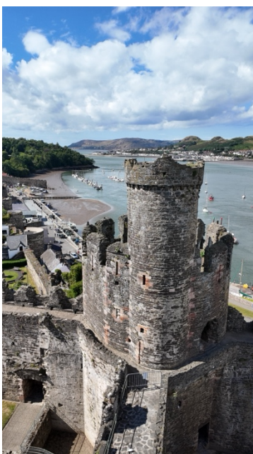
Conwy Castle, Conwy
